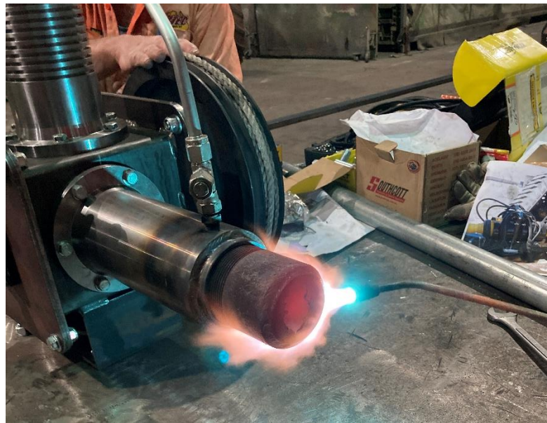
Figure 6.2: Heat being applied to heater head with oxy-acetylene heating torch.
