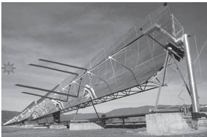
Figure 2.29: Photo of a typical parabolic trough solar collector (Moya 2012).
